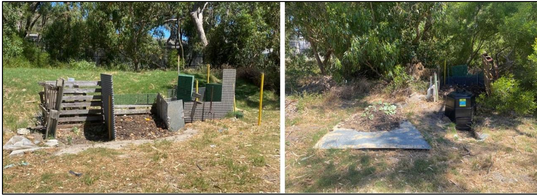
Figure 9. Compost heaps at Wildevoelvlei Water Treatment Plant.
